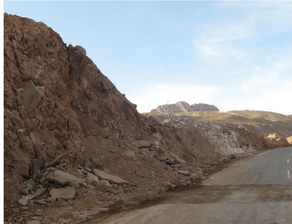
Damage to roads from surface seismic waves (left) and from debris slides (right) as a result of the Nura earthquake (2008)
