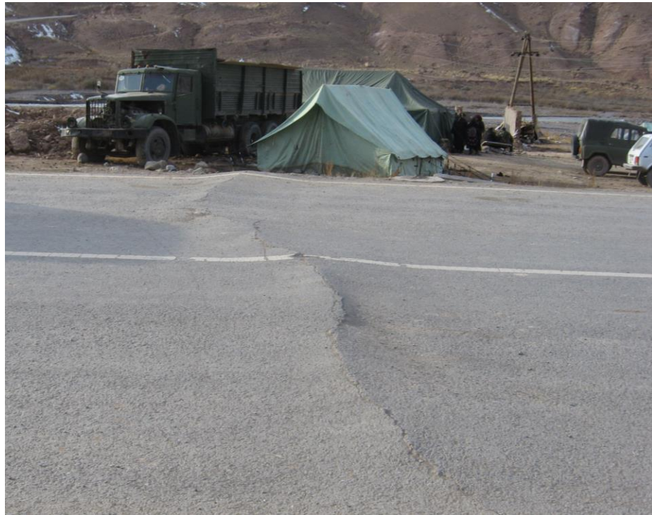
Damage to roads from surface seismic waves (left) and from debris slides (right) as a result of the Nura earthquake (2008)
